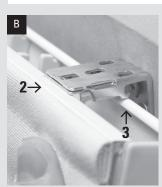
2. Place front lip of internal headbox extrusion on bracket lip by tipping the blind rearward.
