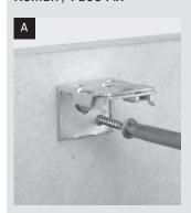
1. Ensure brackets are fitted to desired Face fix position. Ensure brackets are level with each other.
